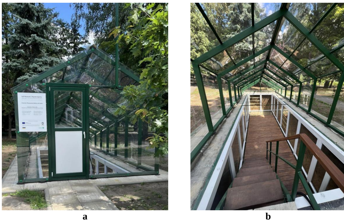
Figure 1. Protective polycarbonate structure over the exposed soil profile on Poltava site: a - outside, b - inside .
