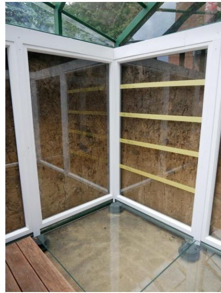
Figure 3. Interior of the shelter, featuring a perimeter ventilation gap and a glazed floor section for observing the parent material
