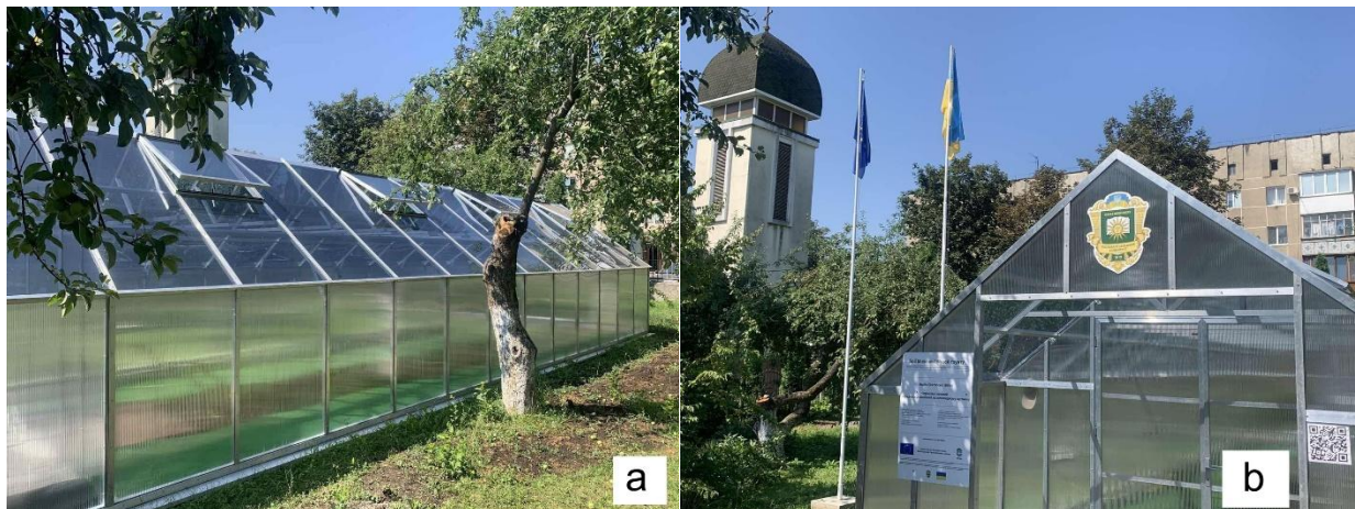
Figure 4. Prefabricated polycarbonate shelter at the Kamianets-Podilskyi site: a- ventilation windows for natural air exchange; b- overview of the museum entrance
